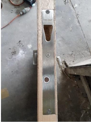
Figure 1 Plate on the door
